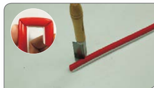
Cut the cover where it is expected to be bent with corner chisel, as shown above.
