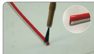
After mounting, cut off excess part of the cover with half round chisel
